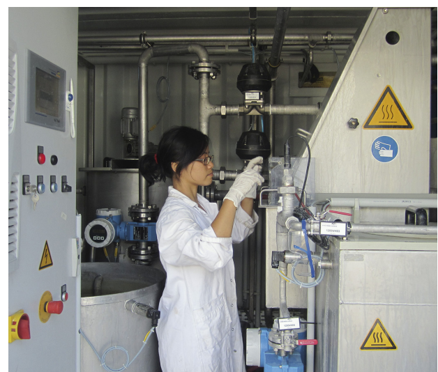
Operation of a pilot plant with membrane technology for the treatment of process waste water of an industrial operation in Vietnam.
